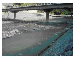
country on October 2005. A former 100 meter long bridge with a 4 meters track that didn't have the right design to cope with floods. It became necessary to design a bridge with the right technical characteristics that took into account the hydrologic studies into account.
