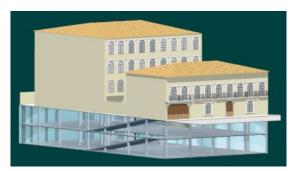
It has spaces for medical services, a pharmacy, a bank office and social events rooms other than the institution offices. The complex has two towers for a total of 3692 square meters and parking space for 55 cars. The building is has a steel structure with concrete blocks walls.
